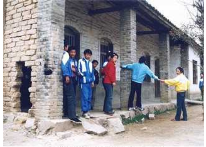
教室断垣残壁,墙体受风雨侵蚀,屋面漏雨
